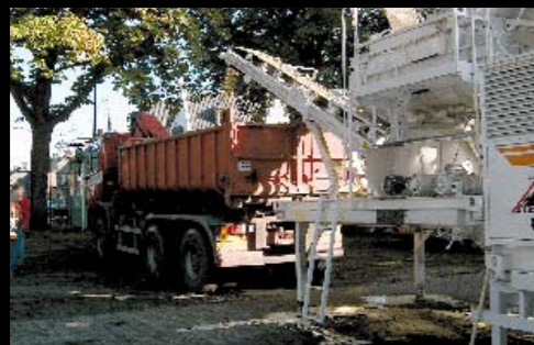
Mix in plant
